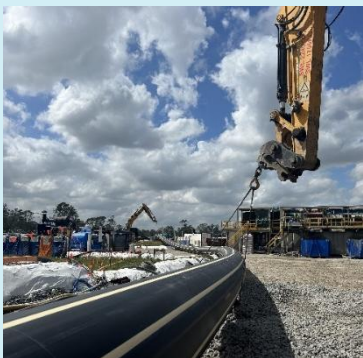
Photo: HDD Installation Gurner Ave, Austral
