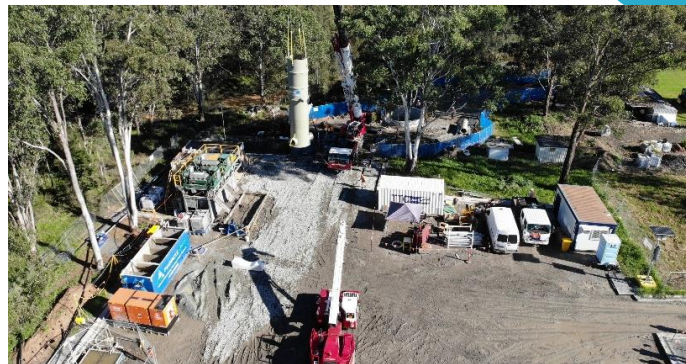
Installation of maintenance hole within private property
