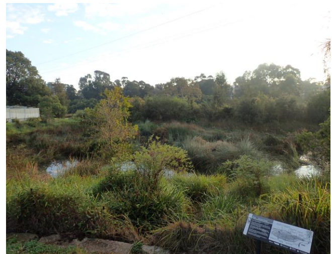
Cup and Saucer Creek constructed wetland in Canterbury treats stormwater runoff from local streets before it enters the Cooks River and has become a thriving wild life habitat area.
