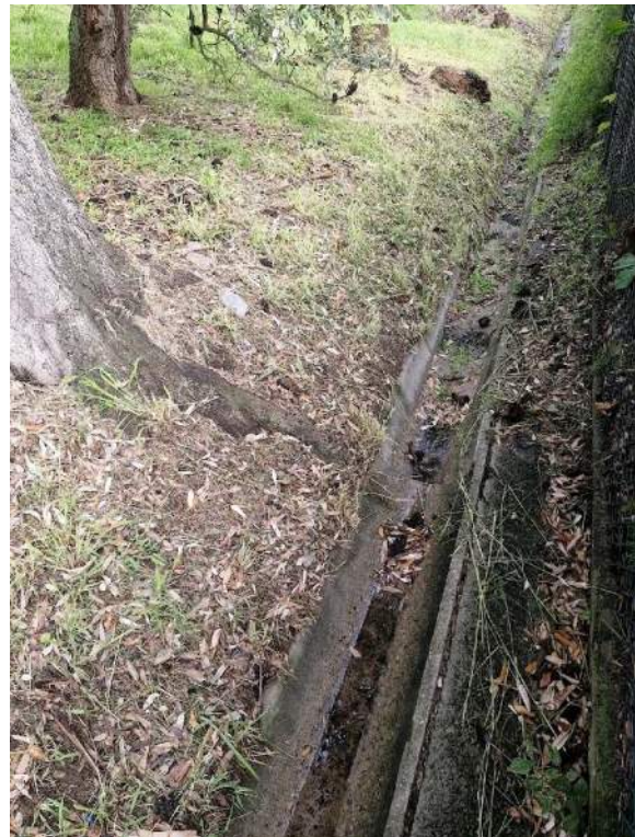
Figure 5: Tree 314 - Structural surface root displacing the adjacent culvert
