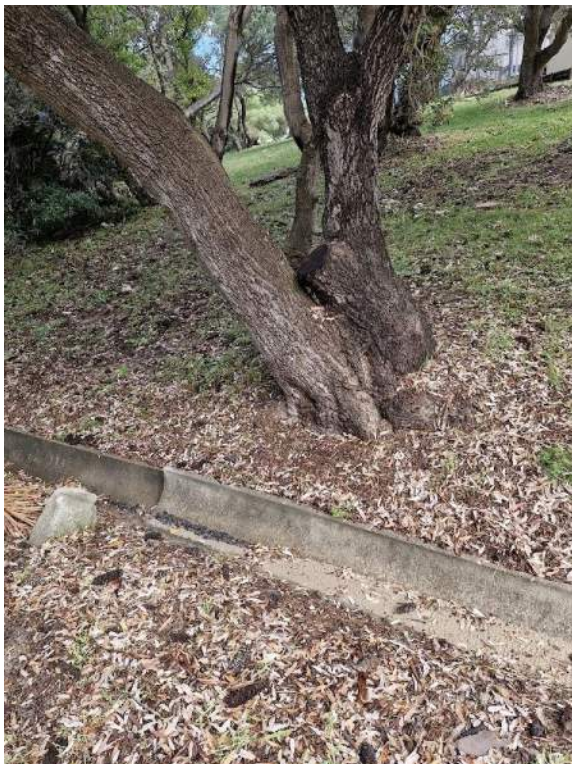
Figure 4: Tree 162 - Within proximity to displaced culvert
