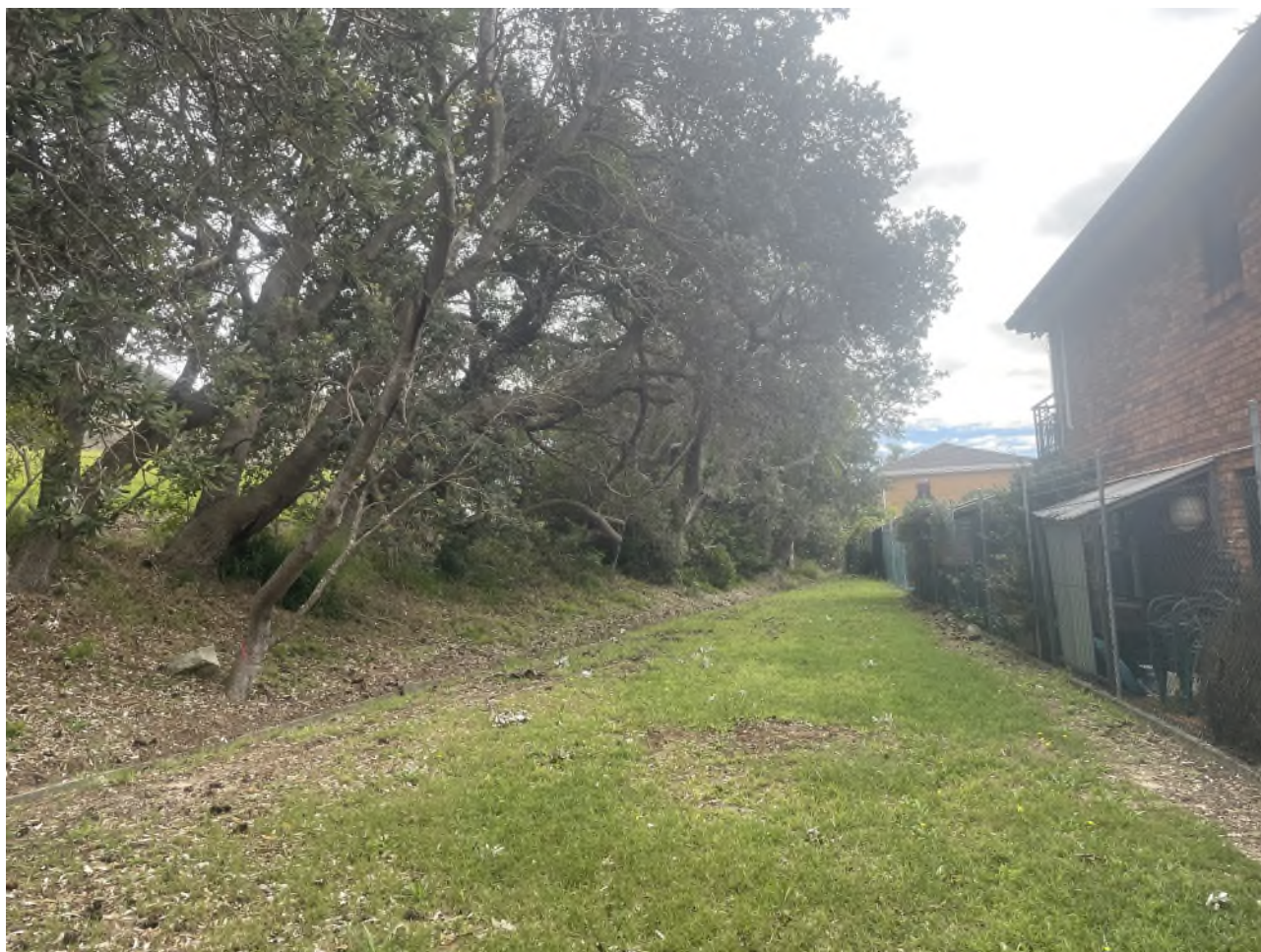
Figure A1: Maroubra Reservoir embankment along the eastern boundary, viewing north and showing vegetation on the embankment that requires removal. Residential properties shown are Fowler Crescent properties.
