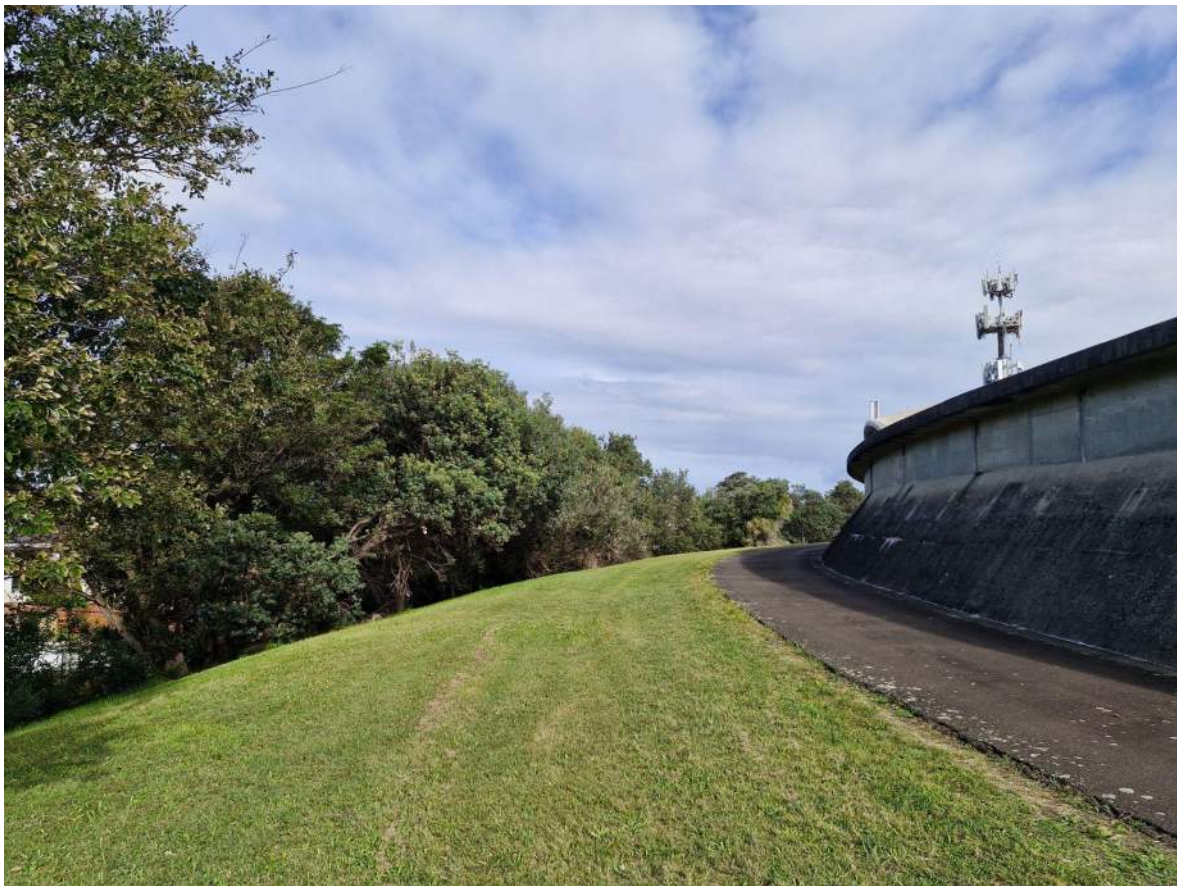
Figure 6: Embankment on the eastern side of the reservoir with non-permitted vegetation (Canopy Consulting, 2024)
