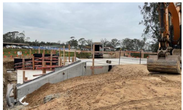
Installed stormwater culvert along Gurner Ave
