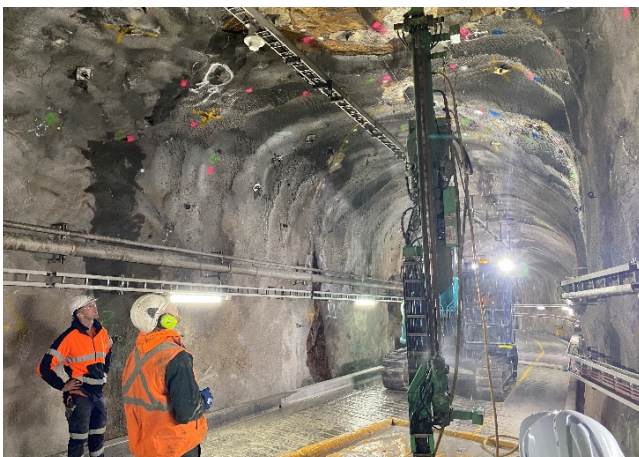
Decline access tunnel repairs
