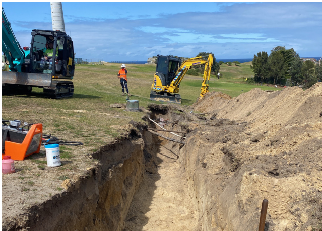
New supernatant pipeline being installed at Bondi Golf Club
