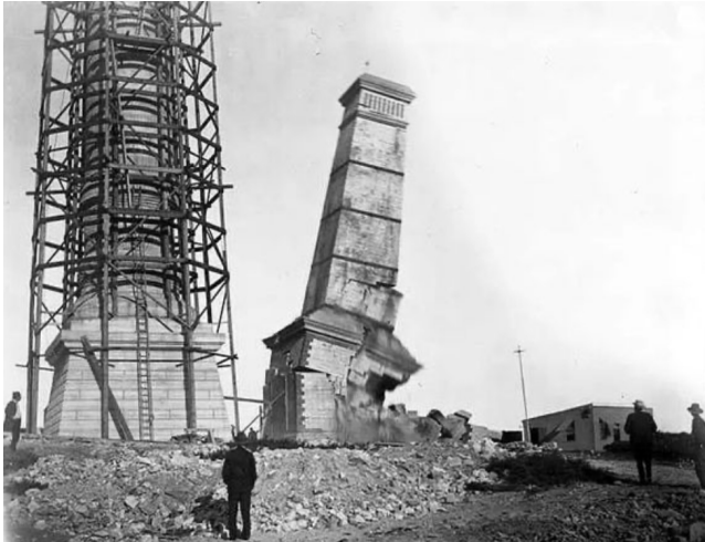
Ben Buckler vent stack being built c.1910 and the original vent stack to the right (Sydney Water archives)
