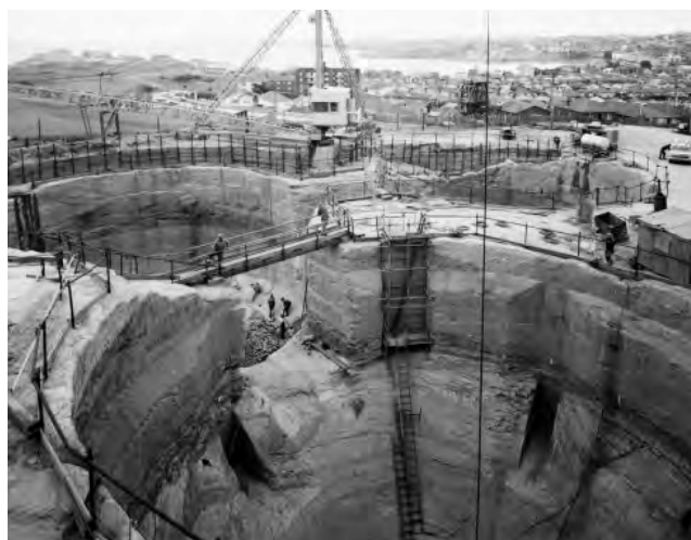
Excavation works for the digesters in the late 1960's. © Sydney Water / WaterNSW Historical Research Archive
