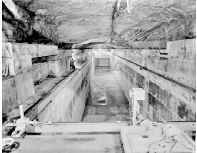
Constructing one of the underground caverns for the sedimentation tanks at Bondi © Sydney Water / WaterNSW Historical Research Archive
