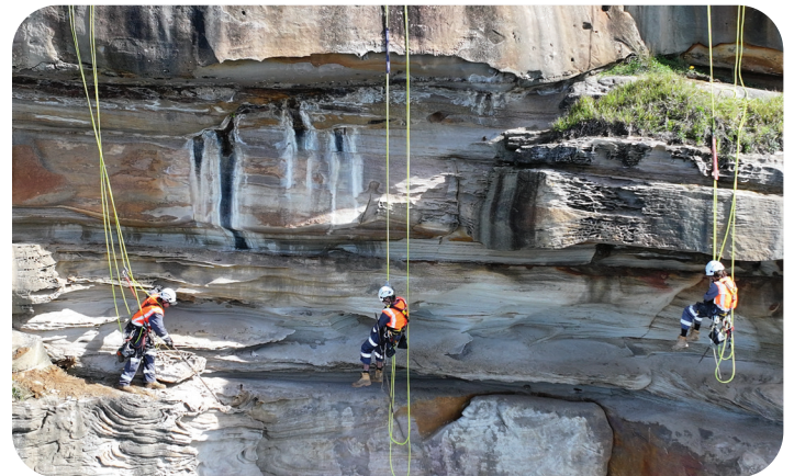
Specialist crews completed structural repairs and safety upgrades to the East Safe Haven emergency exit
