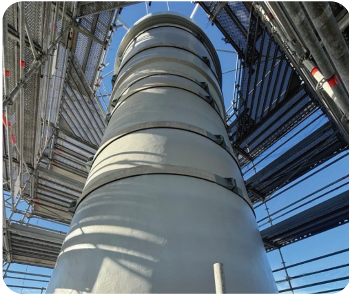
Restoration work on the Ben Buckler stack is helping preserve an important part of Bondi's wastewater infrastructure and local heritage
