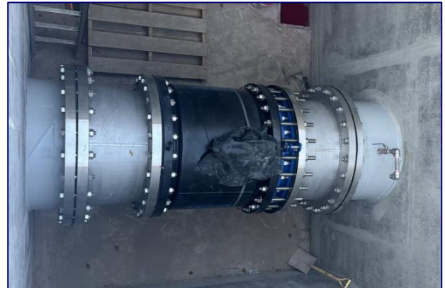
A completed flowmeter connection.
