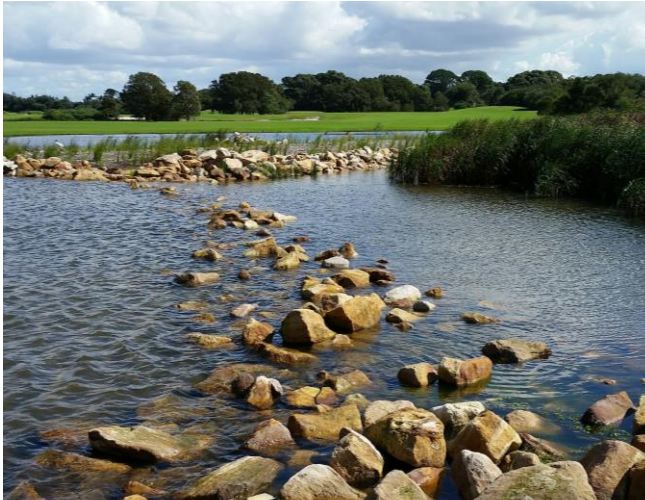
The wetlands at Astrolabe Park act as a natural filter for the stormwater outlet
