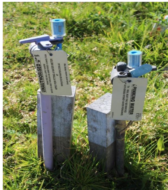
We must install meters going onto these locked and tagged services.
