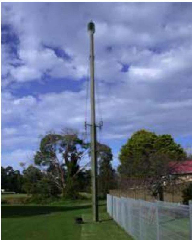
A typical vent shaft in a residential area.
