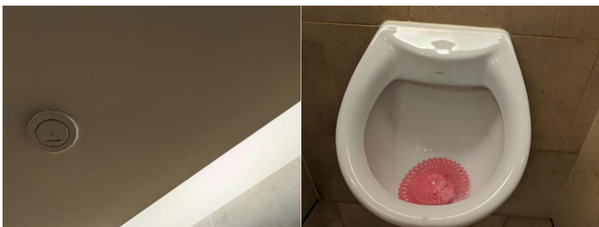
Figure 5-11 Example of Misaligned Urinal Sensor
