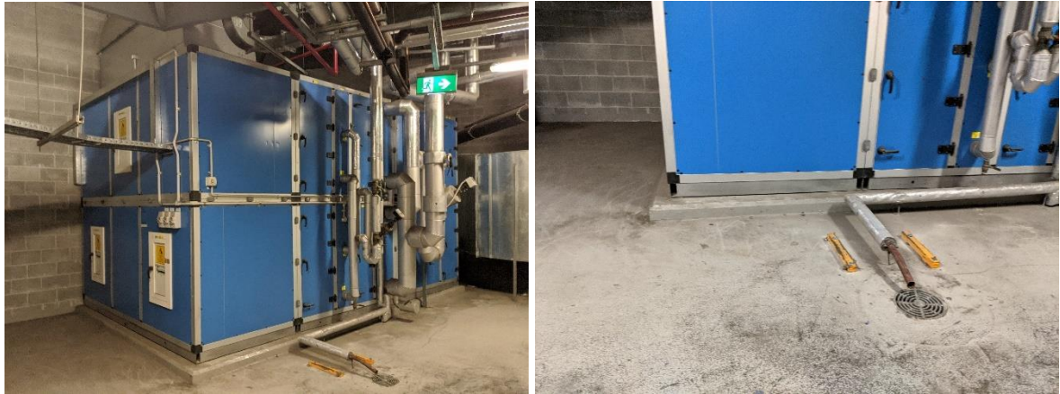
Figure 5-14 Air Handling Unit Condensate Drain Lines
