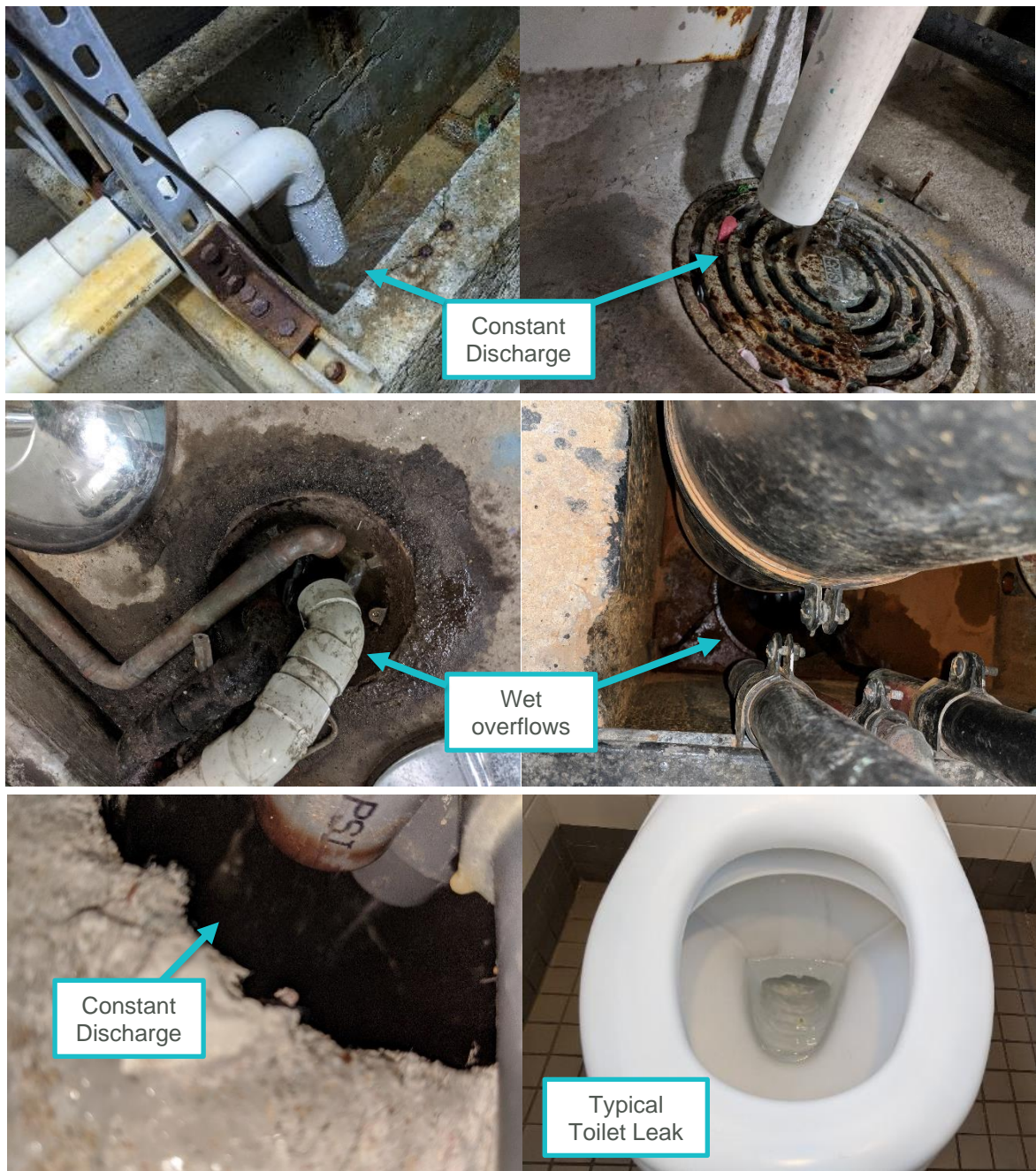
Figure 5-2 Examples of Overflow, Leaks and Losses
