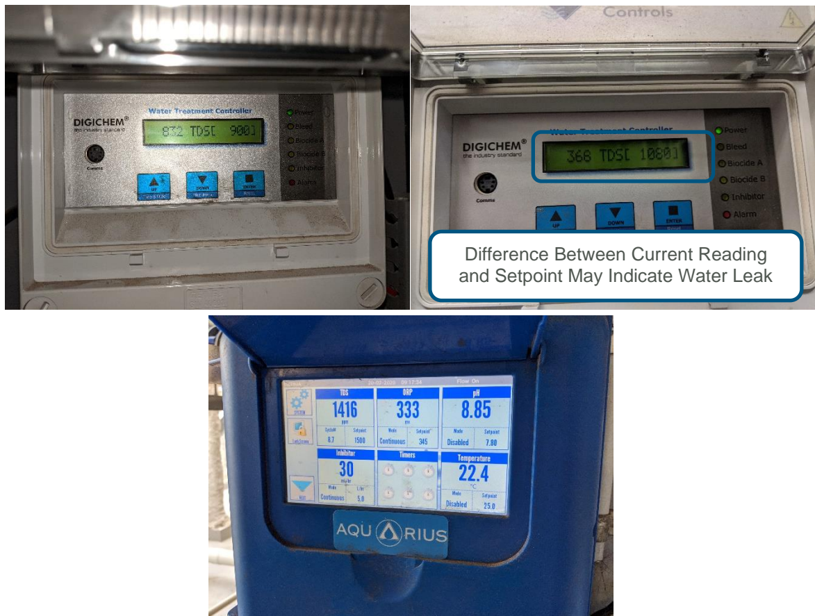
Figure 5-13 Examples of Cooling Tower Control Panels
