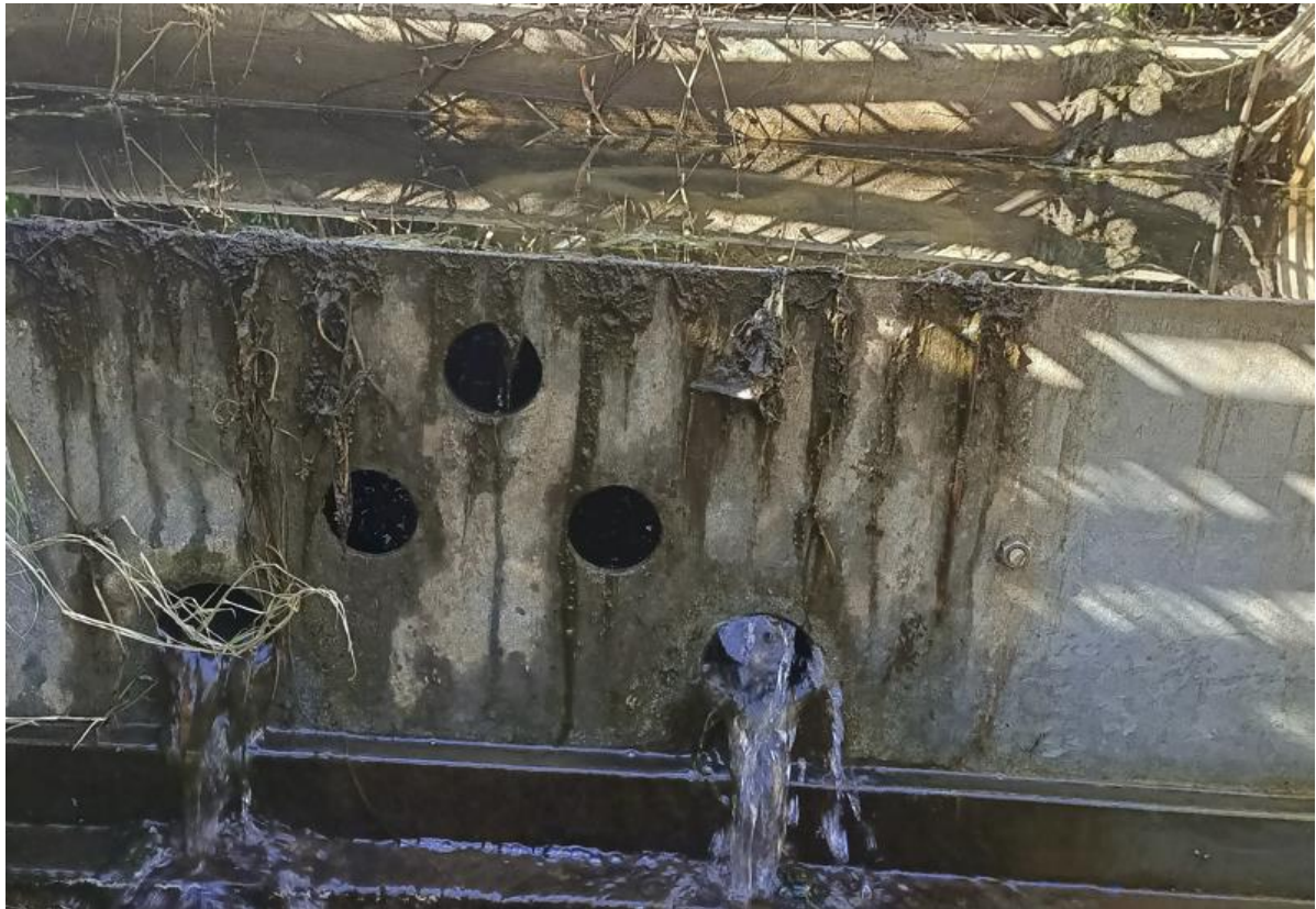
Image 4 holes drilled into stop boards.
