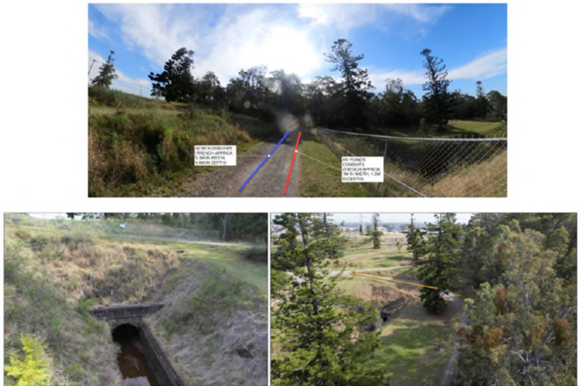
Figure 4-1 Crossing of the Upper Canal System at the Trafalgar Tunnel
