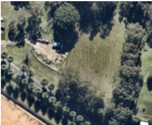
Figure 6: Current (May 2025) condition of Compound 1. Source: SWC Spatial Hub/NearMap.
