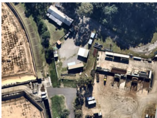
Figure 8: Current (May 2025) condition of Compound 2. Source: SWC Spatial Hub/NearMap.
