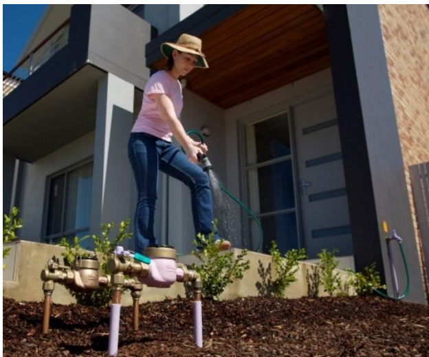
Recycled water pipes, taps and meters are coloured purple to distinguish them from the drinking water system.
