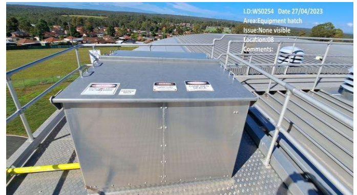
Access with equipment hatch
