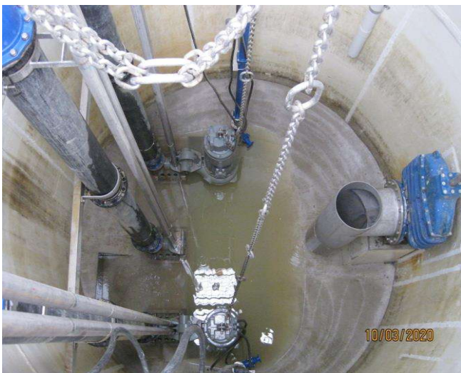
Marsden Park SP1173 wet well – Capacity 330 l/s
