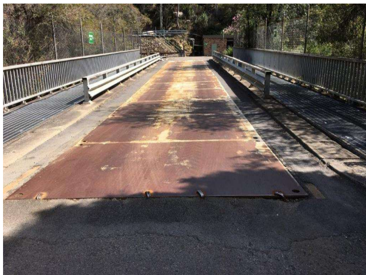
Existing bridge crossing
