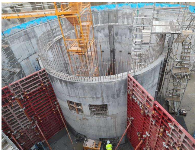
Construction of Northmead SP1220 – Capacity 840 l/s
