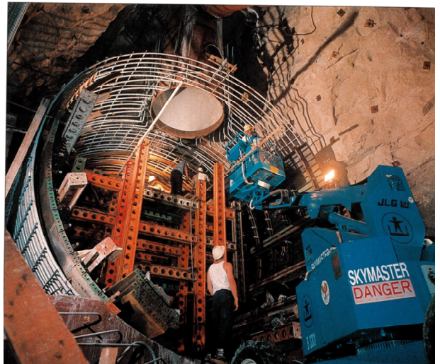
Erecting formwork for de-aeration chamber
