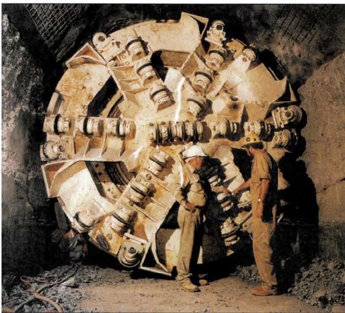
Tunnel Boring Machine used in DOOF Construction
