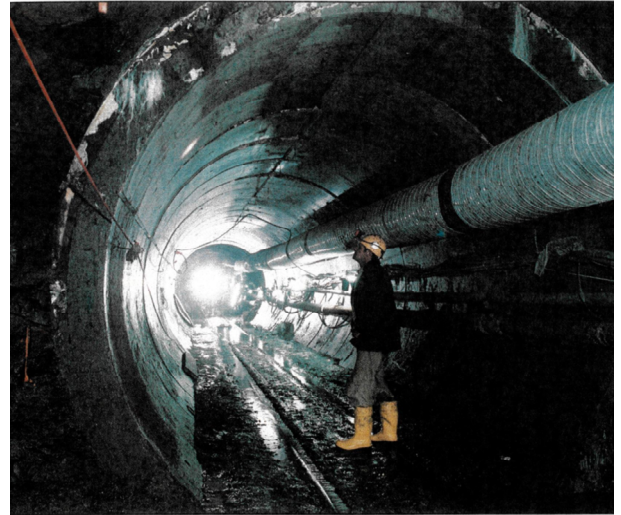
Inspecting Pre-cast Lining in DOOF Tunnel
