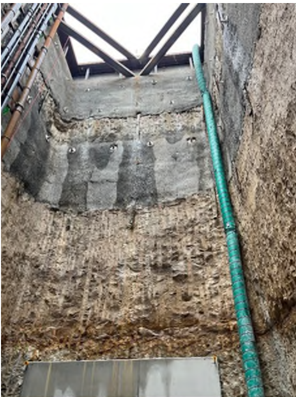
Launch Shaft at Lot 96
