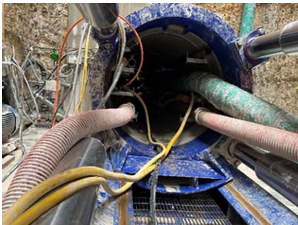
Tunnelling being carried out from Lot 96 towards SP1022
