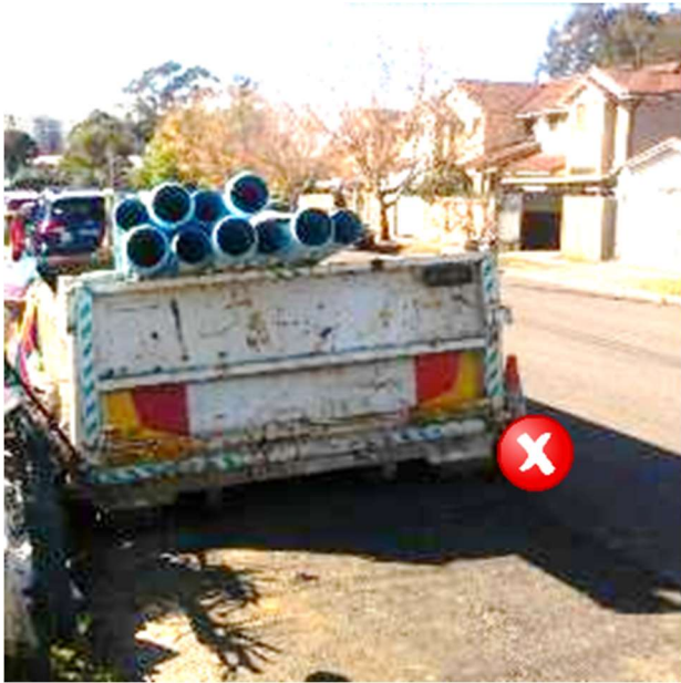
Figure 3 Pipes stored without protective caps
