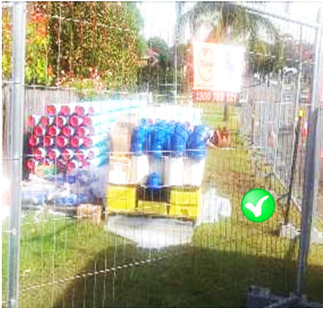
Figure 4 Pipes and fittings stored with protective caps
