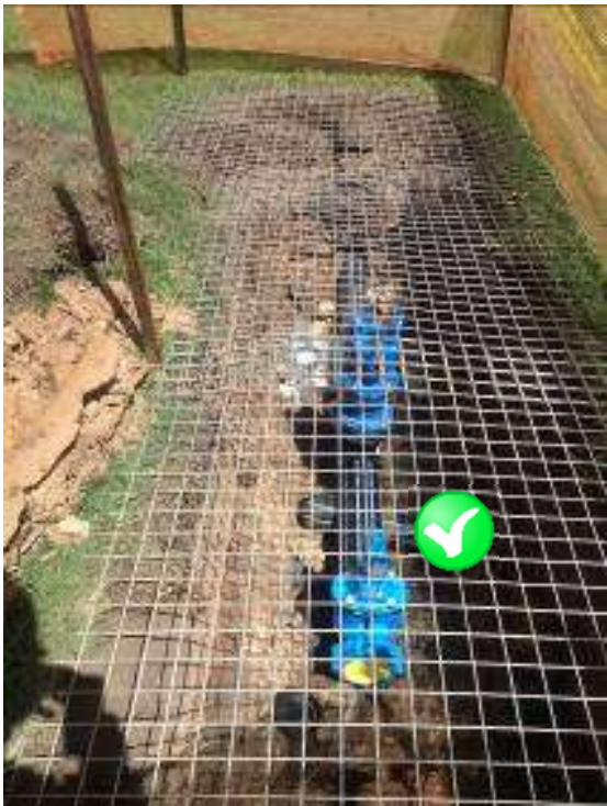
Figure 2 Fittings capped overnight in trench
