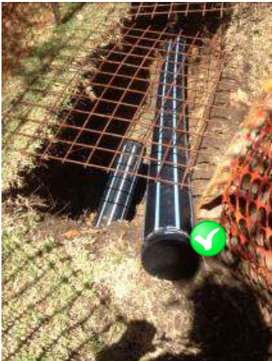
Figure 1 Pipes capped overnight in trench
