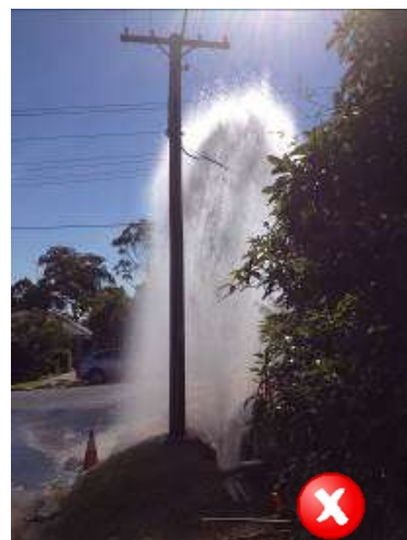
Figure 7 Discharged water & swab uncontrolled
