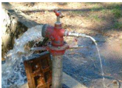
Figure 10 Standpipe with sampling tap
