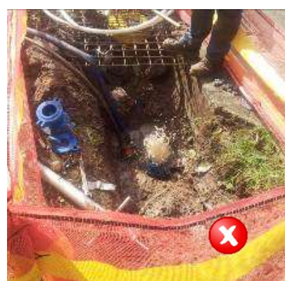
Figure 7 Discharged water & swab uncontrolled
