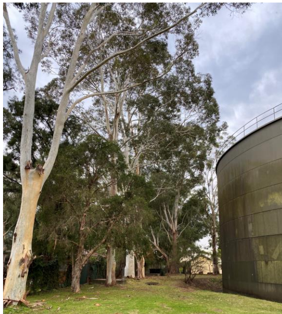
Figure 6-1 Photo of the site including existing reservoir
