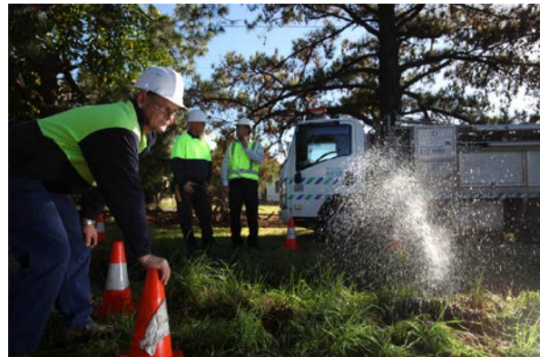
A Sydney Water crew fixing a water main break.
