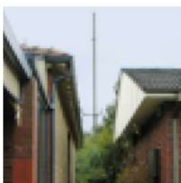
Sewer Vent Shaft
