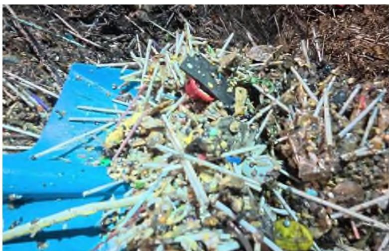
Figure 46: Material removed from behind the North Head bulkhead door
