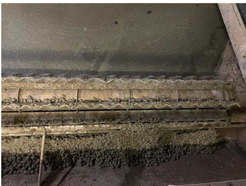
Figure 21: Debris balls captured in the scum systems of PST1 and PST2 on 1 July 2025.
