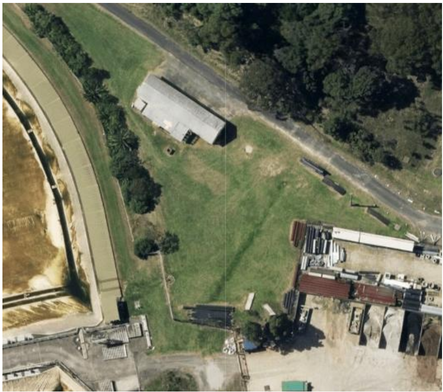
Figure 7 Former (2021) condition of Compound 2
