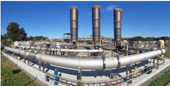
Figure 3 Waste Gas Burner Pipework Upgrades
