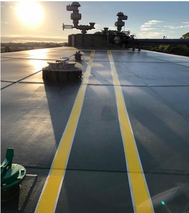
Figure 1 Refurbished roof of cleaned and almost finished 3rd digester
