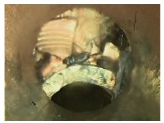
Example of clear photo evidence showing displaced and collapsed pipework at the end of a section of pipe.
