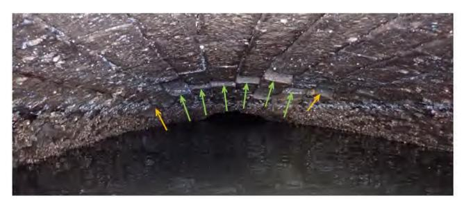
Figure 1 Example of sections in poor conditions (arch deformation and block displacement)
