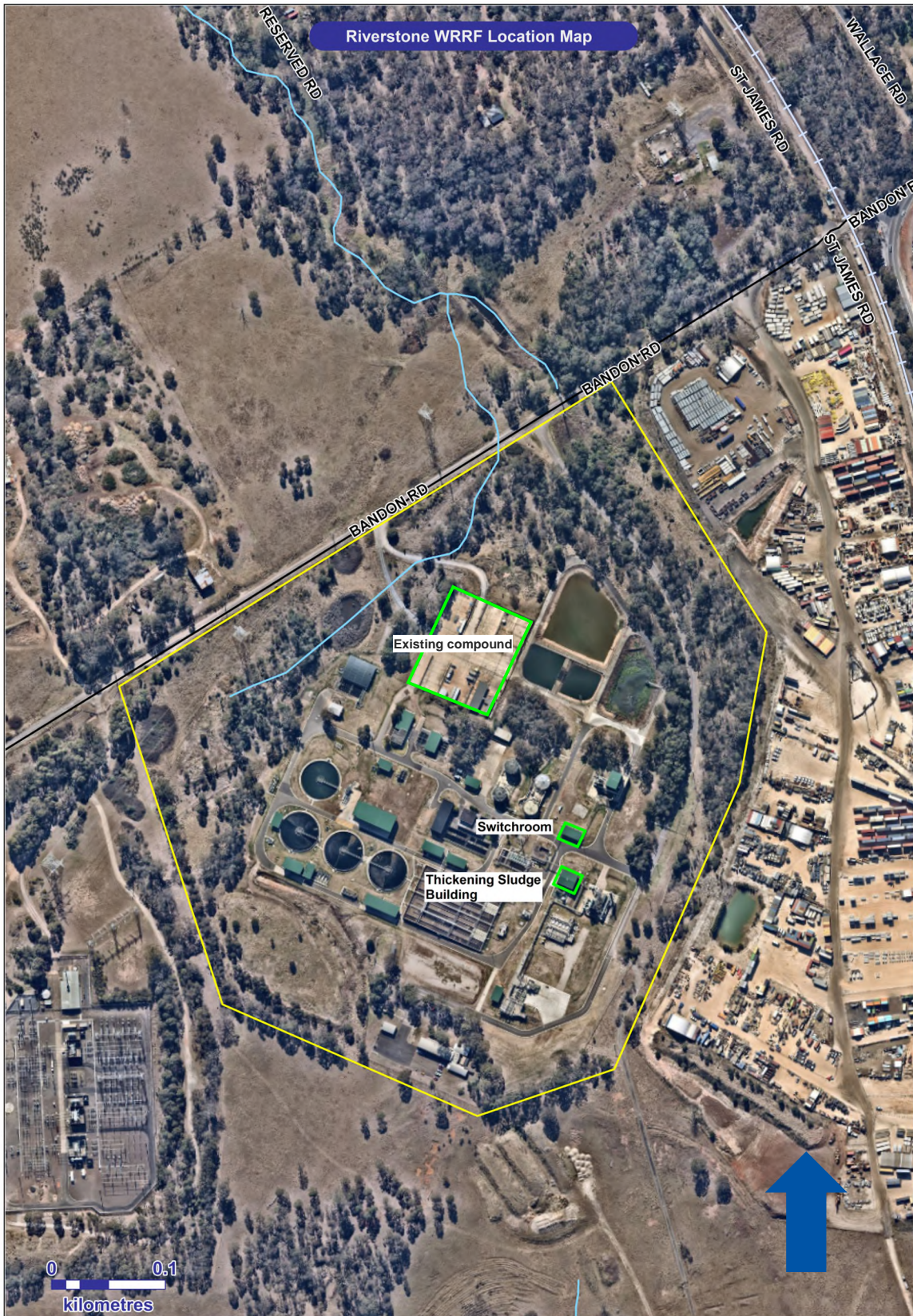
Figure 1 Location of proposal (all works contained within the existing thickening sludge building with exception of VSD installation at the switchroom. Riverstone WRRF boundary indicated by yellow line)
