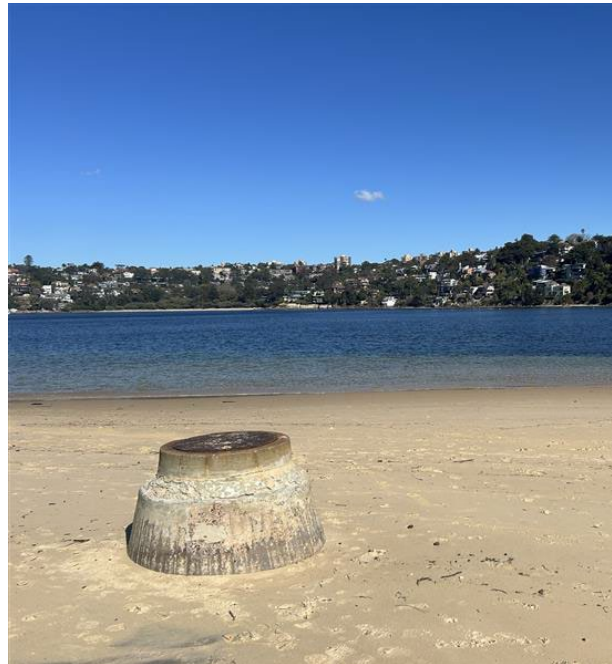
Plate 4: Concrete maintenance hole on foreshore
