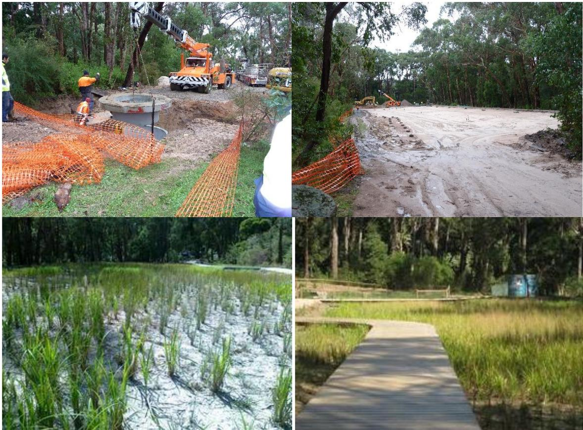
Figure 3 The Wicks Reserve Biofilter (a) GPT installation, (b) Biofilter construction, (c) establishment, (d) established, Sources (a) and (b) Dale Browne, (c) and (d) Clearwater case study (Clearwater, 2012)
