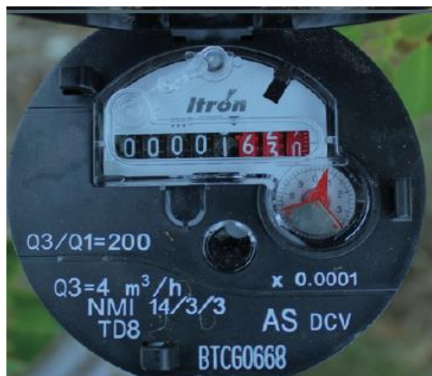
Use the water meter to check for leaks at any time.
