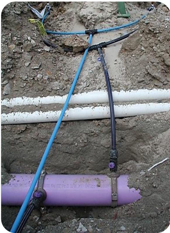
Recycled water is supplied through a pipeline that is separate to the drinking water pipe
