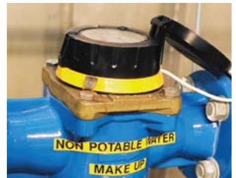
Top: AstraZeneca's Engineering Manager – Facility Services, Mike Crompton and Sydney Water's Project Officer, Carl Binns inspect the Nova facility's non-potable process water tank.
