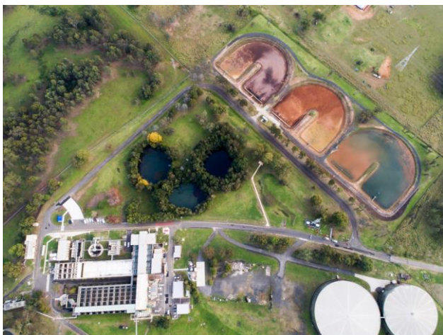
Orchard Hills Water Filtration plant
