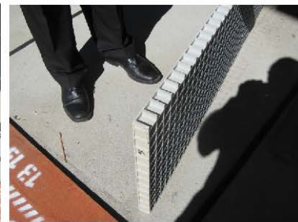
FIGURE 4 – INLET WORKS COVERS FIGURE 5 – INLET COVER PANEL
