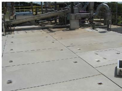
FIGURE 6 – INLET WORKS COVERS FIGURE 7 – INLET COVER PANEL
