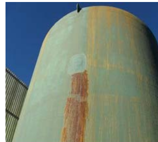
Fractured laminate
