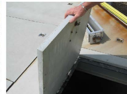
FIGURE 6 – INLET WORKS COVERS FIGURE 7 – INLET COVER PANEL
