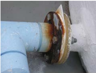
Blister and delamination of pipe flange
