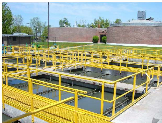
FIGURE 18 - SEDIMENTATION TANKS GRATING
