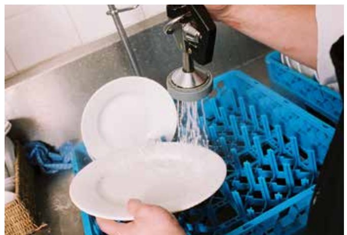
Using water-efficient smart rinse valves is one way you can save water.
